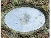
3 - Place the base plate on top of the anchor ensuring the bolt holes line up.
